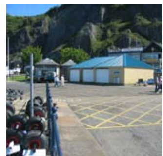
Existing facilities, Knab Rock
